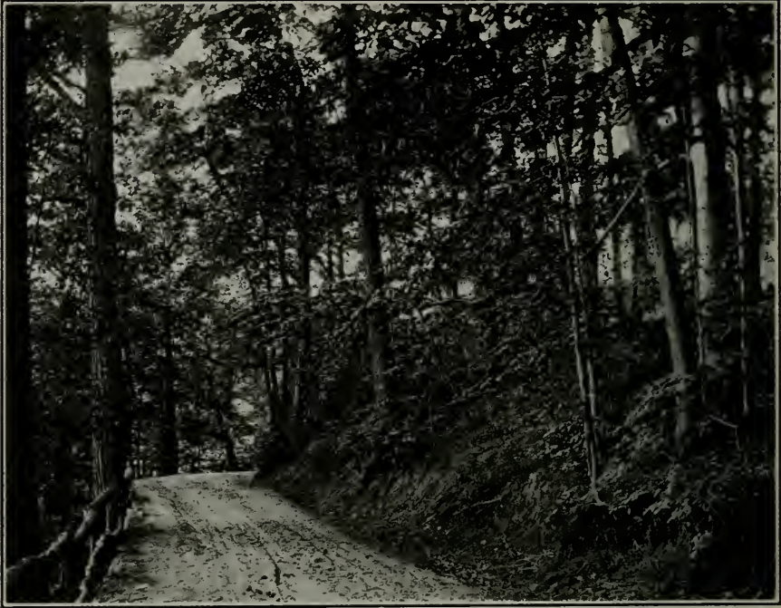
DRIVEWAY IN "ROCKRIMMON" ESTATE."
